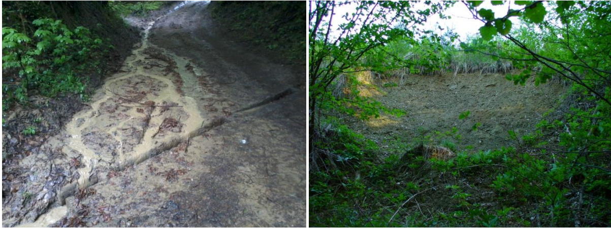
Figure 1.7. Erosion processes in forested catchments: soil loss from an unpaved forest road (left) and mass movement (right) (Sopron Hills)
